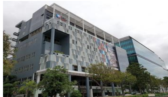
GPS Office at Tai Seng Street
